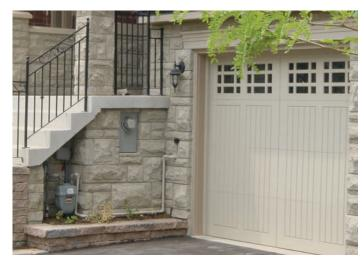
For Townhouses and other higher density forms, utility meters should be architecturally integrated or screened
