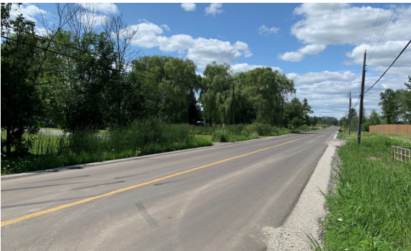
Figure 14 - West Site Image
