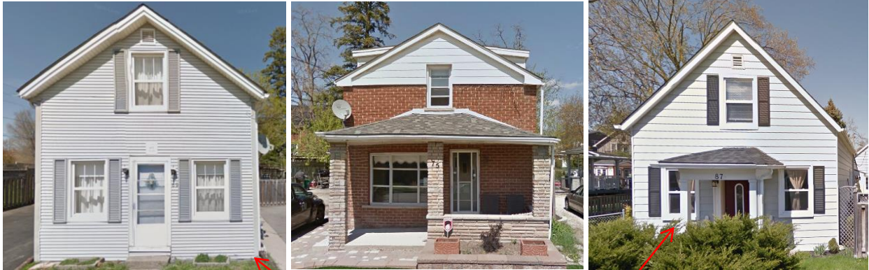
69, 75 and 87 Commercial Street
