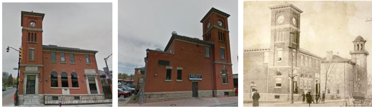
Milton former Post Office 2009 and c.1916
