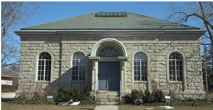
Former Halton County Registry Office, King Street (1915)
