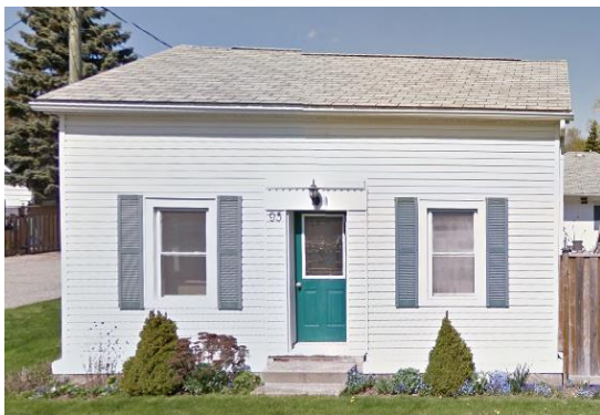
Robert Wales House, 95 Commercial Street
