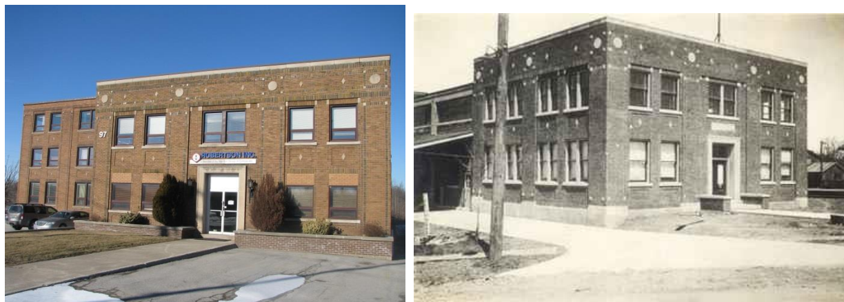
Former Robinson Screw Factory Building 2015 and c.1930
