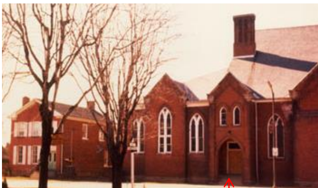
St. Paul's Church c.1950 (prior to construction of Christian Education Centre). The western end of the church is the 1852 structure.
